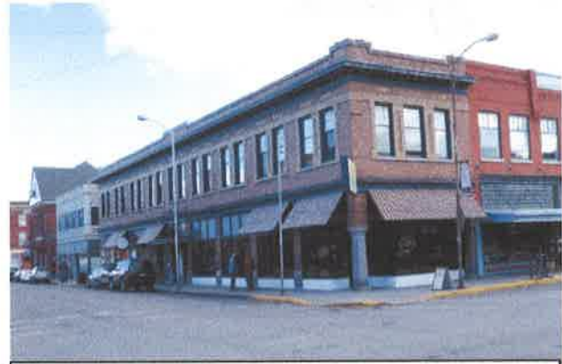
Photo #1: 101 S. Main & W. Callender St. Building
