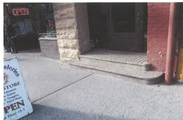
Photo #2: Stair at Callender St. Entry
