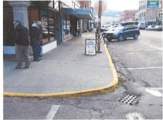
Main St. Surface View
