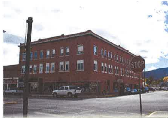
Photo #1: 206 Main & Lewis Street
