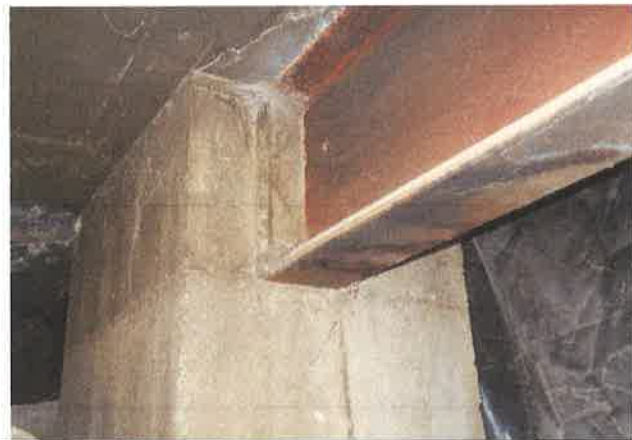
Photo #2: Building Line Steel Bm & Conc Column
