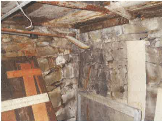
Stone Rubble End Wall & Building Foundation
