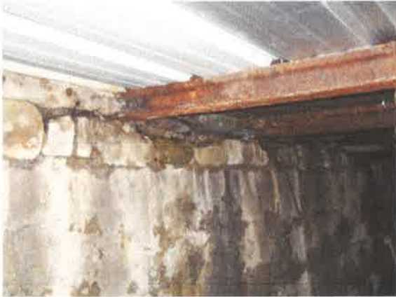
Street Side Foundation Wall & Vault Lid
