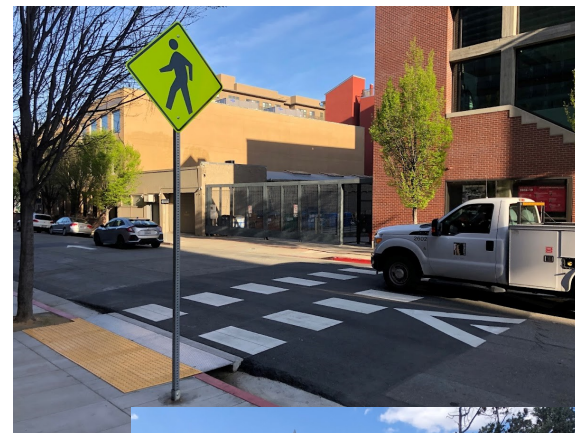
Mid-block raised crosswalk examples showing a bridging of the gutter (top) and in combination with a curb extension (middle).
