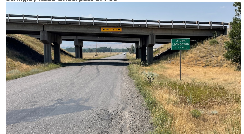
Swingley Road Underpass of I-90
