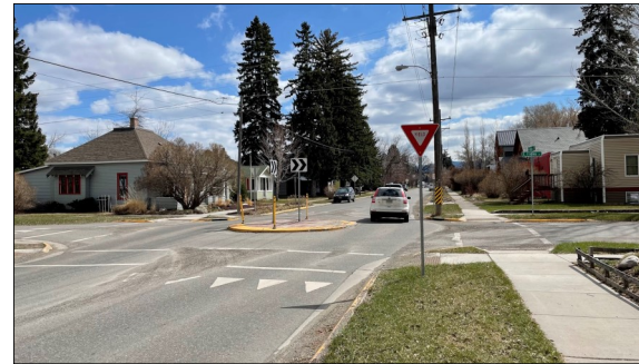
Mini-roundabouts on Wallace St in Bozeman (left) and Wyoming St in Missoula (below).
