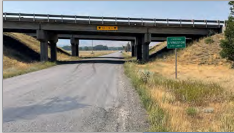
Meyers Lane Underpass
