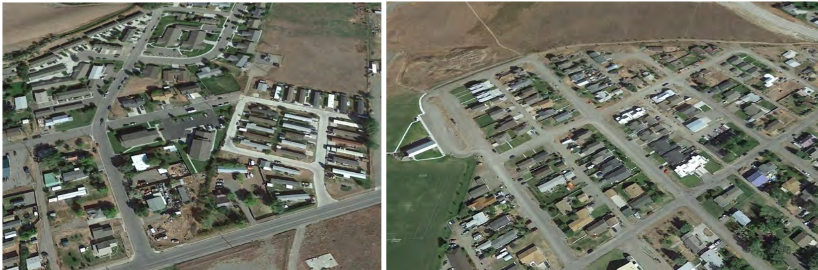
Figure 7-2: Recent Developments or Individual Parcels Lacking Sidewalks
