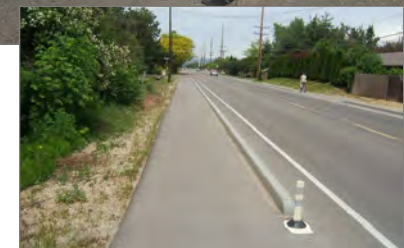
An expanded shoulder with an extruded curb walking on the north/east side may be a short-term option from Miles Street to Park Street.
