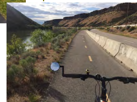
Sidepath with Vertical Barrier
