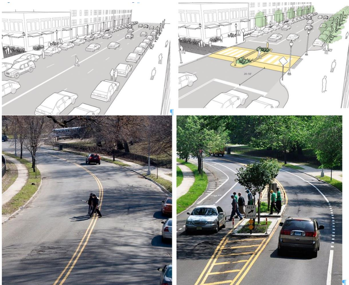
Figure 9 Before and after midblock crossing infrastructure
