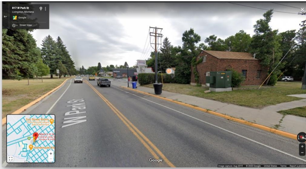
Figure 5 Marks In and Out/NWE building and Park Street Intersection (Source: Google)
