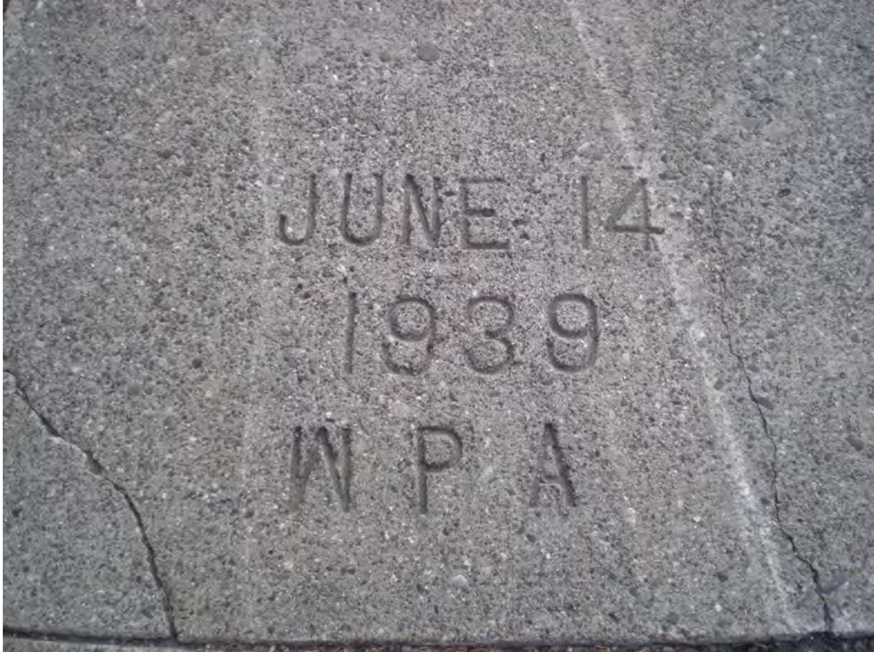
MT_ParkCounty_Sacajawea/Miles Park Historic District_0026 Yellowstone River Bridge (Resource #2) stamp on northeast sidewalk.
