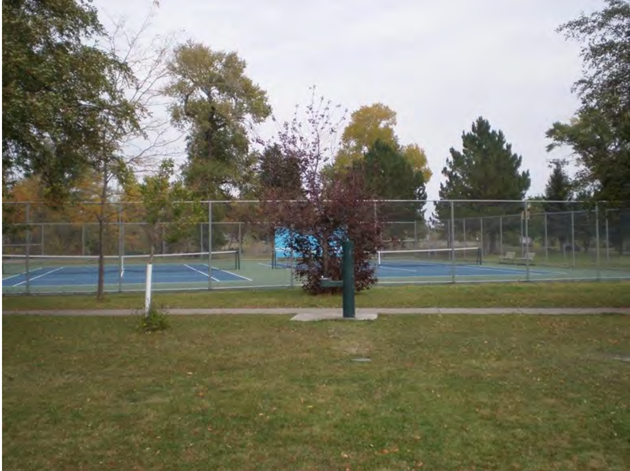
MT_ParkCounty_Sacajawea/Miles Park Historic District_0006 Two WPA-era Tennis Courts (Resource #1) in Sacajawea Park area of Sacajawea/Miles Park Historic District. View to the south from McGee Drive.
