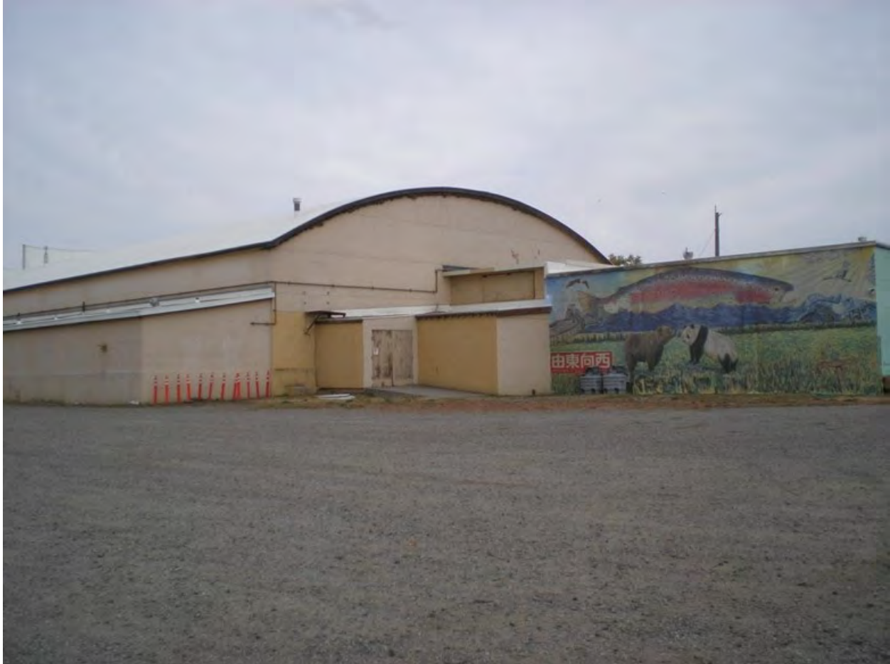
MT_ParkCounty_Sacajawea/Miles Park Historic District_0042 Armory/Civic Center (Resource #21) showing rear additions [west and south walls of main block and west walls of additions]. View to the north from gravel parking lot.
