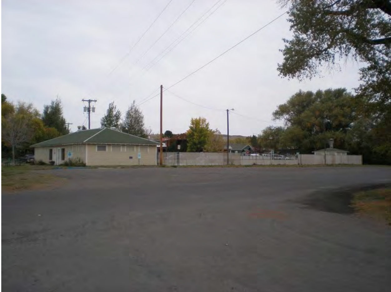
MT_ParkCounty_Sacajawea/Miles Park Historic District_0035 Office/Bathhouse (Resource #24) [west and south walls], City Swimming Pool (Resource #23), and Pump House (Resource #25) [west and south walls]. View to the north across River Drive toward South 2 nd Street.
