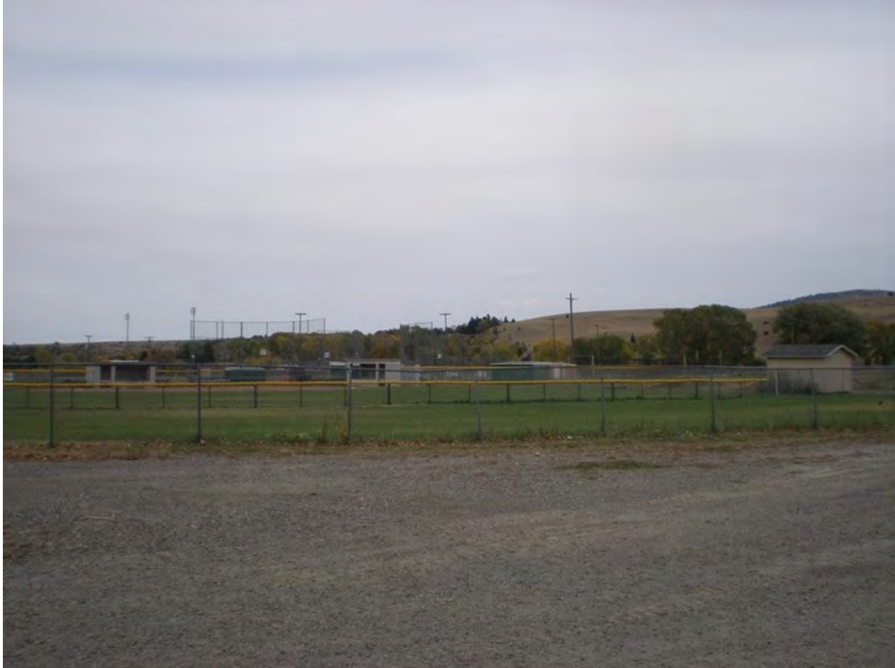
MT_ParkCounty_Sacajawea/Miles Park Historic District_0034 Baseball Fields (Resource #29). View east across the Armory/Civic Center gravel parking area, Miles Park portion of the Sacajawea/Miles Park Historic District.
