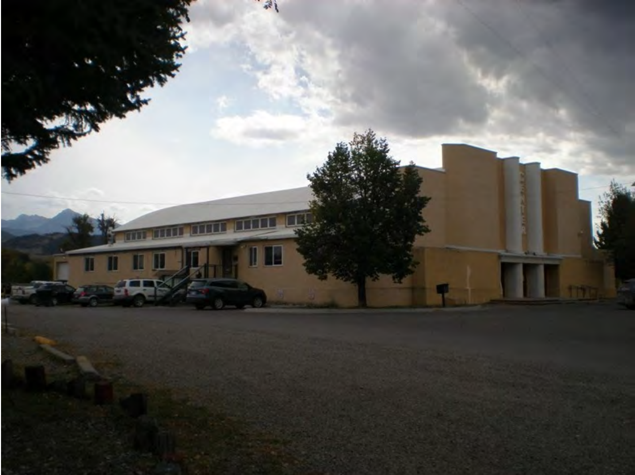
MT_ParkCounty_Sacajawea/Miles Park Historic District_0041 Armory/Civic Center (Resource #21) [east wall and north facade] in Miles Park portion of Sacajawea/Miles Park Historic District. View to the south from River Drive.
