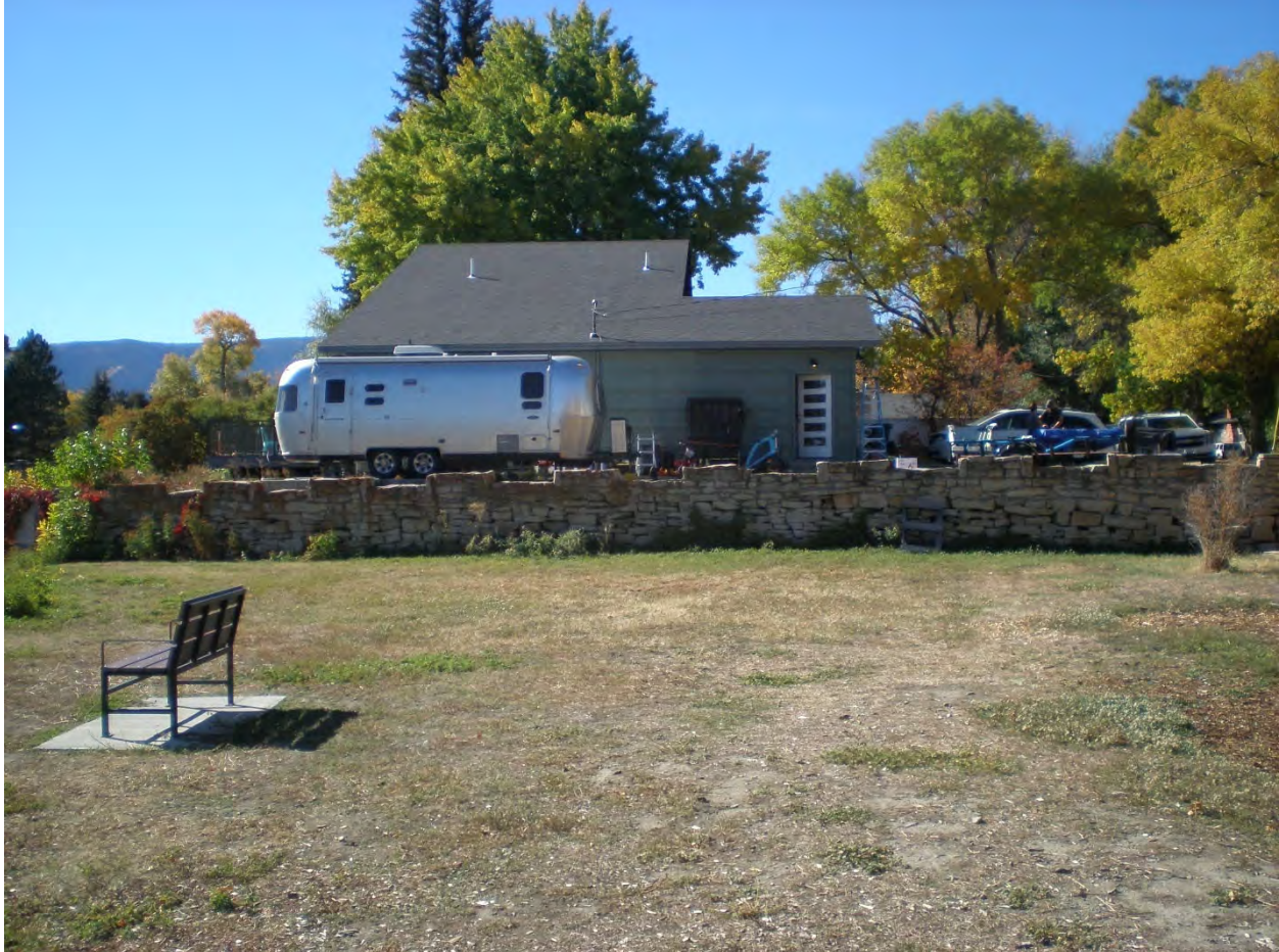
MT_ParkCounty_Sacajawea/Miles Park Historic District_0062 Stone Wall (Resource #36) bounding west edge of Fireman's Park. View to the west from Climbing Stones.
