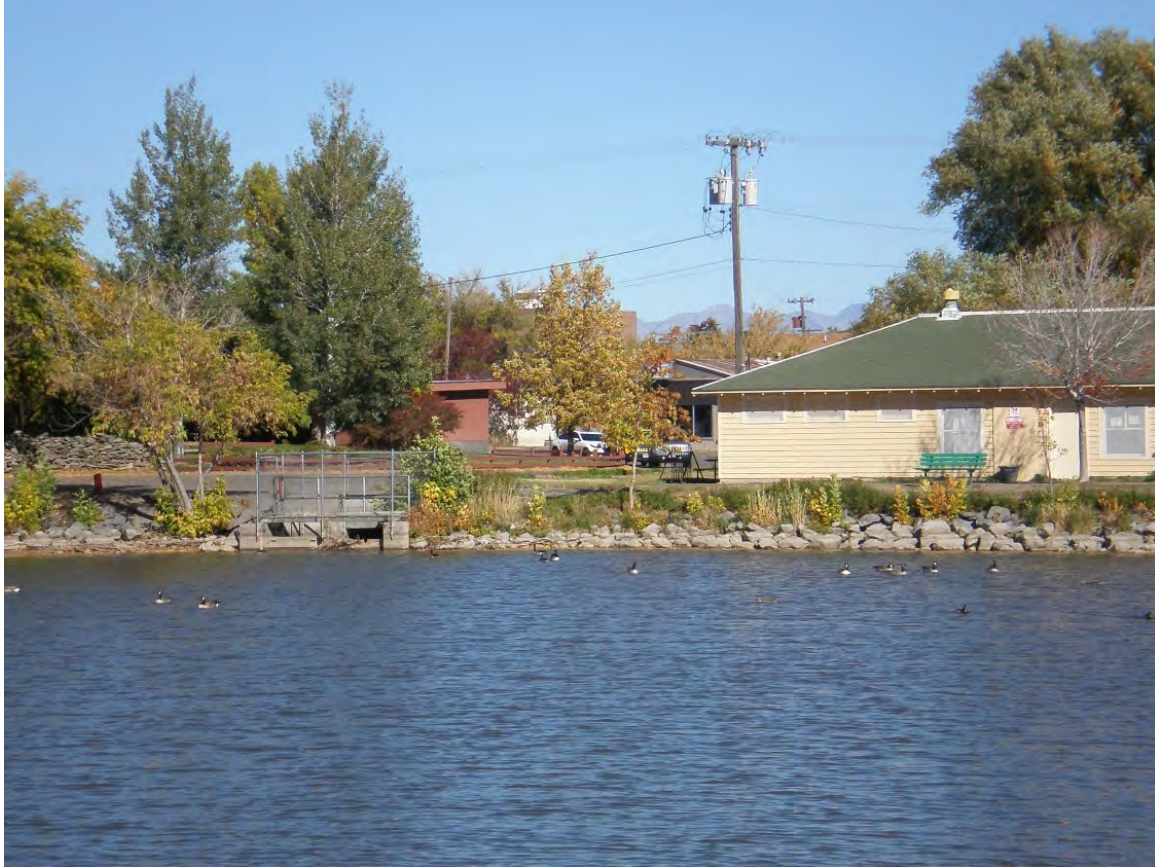
MT_ParkCounty_Sacajawea/Miles Park Historic District_0038 Eastern-most WPA-constructed dam (Resource #27) and Office/Bathhouse (Resource #24) [west wall] with dam weir on left side of image. View to the east from River Drive.
