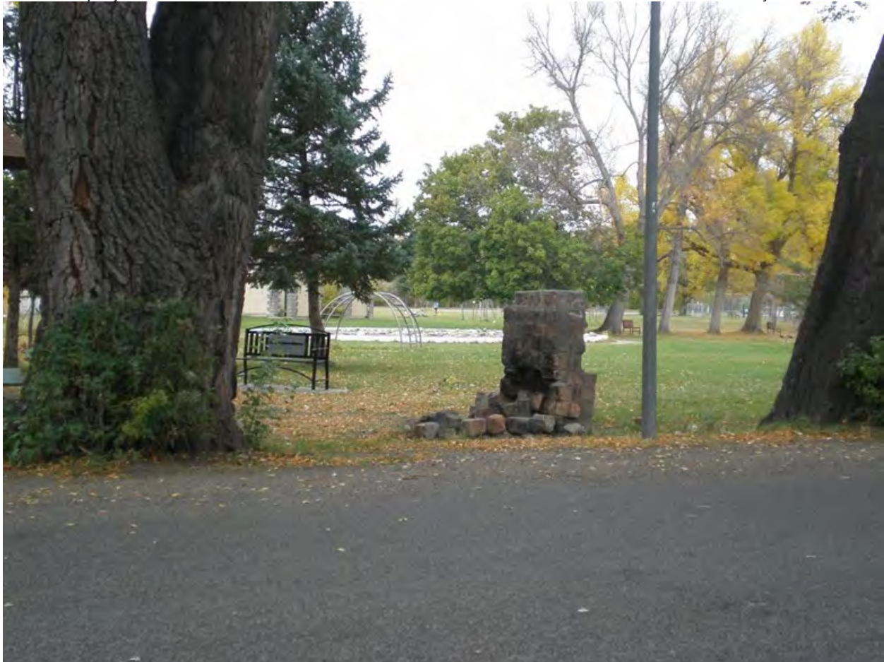
MT_ParkCounty_Sacajawea/Miles Park Historic District_0005 Barbecue (Resource #5) with Wading Pool (Resource #6) in the background, Sacajawea Park area of Sacajawea/Miles Park Historic District. View to the north from River Drive.
