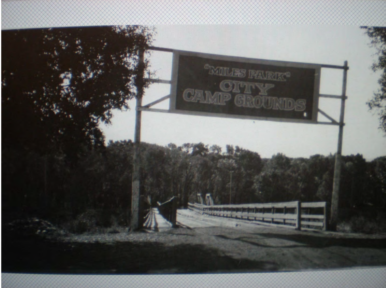
Undated photograph looking south across the west channel of the Yellowstone River near the bridge on 2nd Street. View toward McLeod Island.
