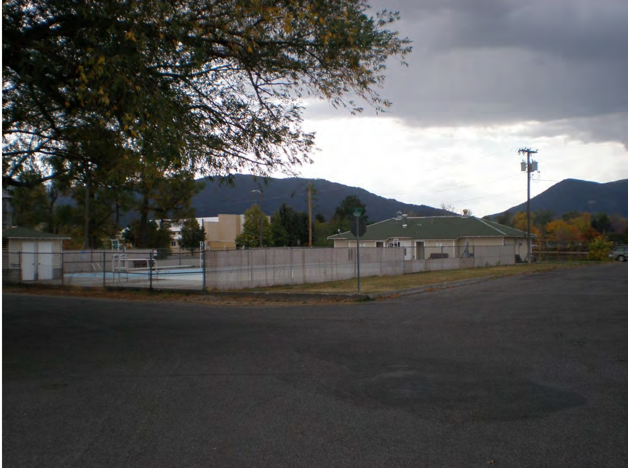
MT_ParkCounty_Sacajawea/Miles Park Historic District_0037 Overview of Pump House (Resource #25) [north wall], City Swimming Pool (Resource #23), and Office/Bathhouse (Resource #24) [east and north walls] in background. View to the southwest across 2nd Street from intersection of West Butte Street and South 2 nd Street.
