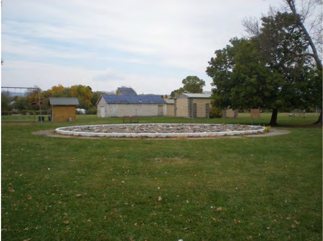
MT_ParkCounty_Sacajawea/Miles Park Historic District_0004 Wading Pool (Resource 6) and park department storage buildings (Resources #7, 9, 10, 11), southeast area of Sacajawea Park area of Sacajawea/Miles Park Historic District. View to the northwest from River Drive.
