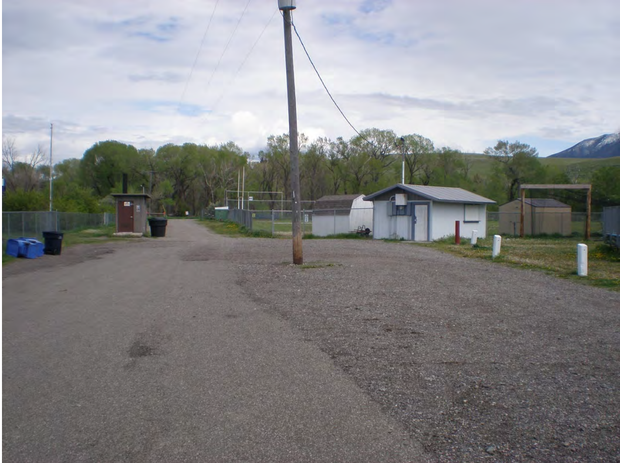
MT_ParkCounty_Sacajawea/Miles Park Historic District_0053 Electrical Shed (Resource #31), south end of the Baseball Fields (Resource #29) with one of six Modern Sheds (Resource #30) to the immediate left and one of six Vault Toilets (Resource #18) to far left. View to the east.
