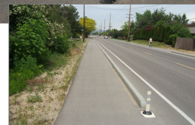
An expanded shoulder with an extruded curb walking on the north/east side may be a short-term option from Miles Street to Park Street.
