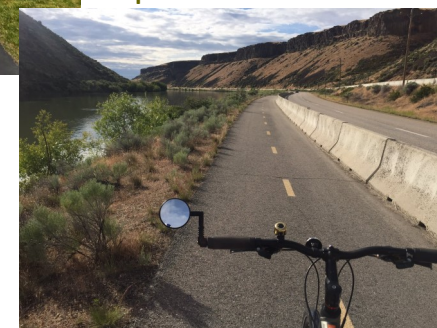
Sidepath with Vertical Barrier
