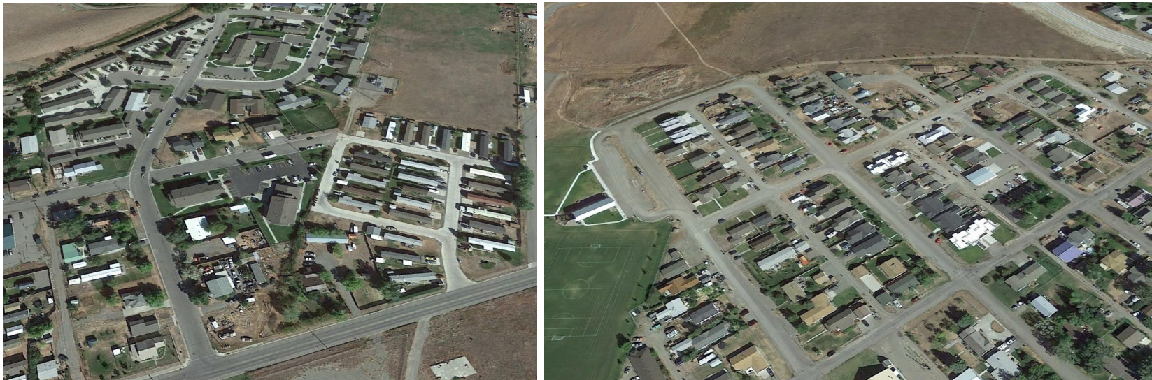
Figure 7-2: Recent Developments or Individual Parcels Lacking Sidewalks
