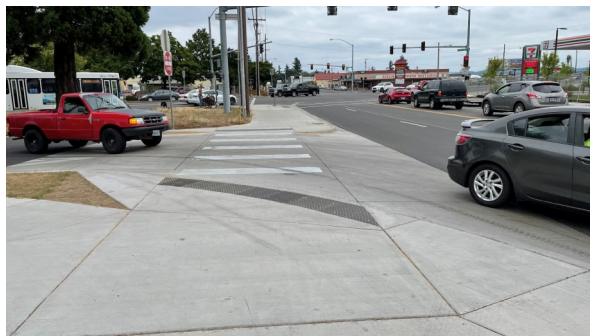
Raised crosswalks at a shared use pathway crossing of a right turn slip lane.
