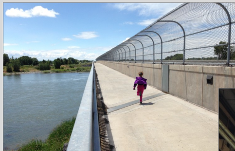
Shared Use Pathway alongside I-15 over the Snake River in Blackfoot, ID.
