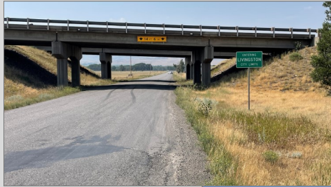
Meyers Lane Underpass
