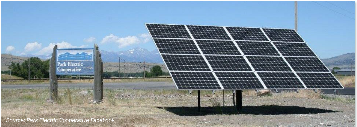
Figure 9.1: Park Electric Cooperative
