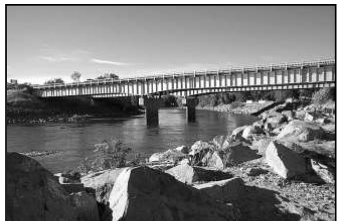
Photo 13. Interstate 90 Bridge. Photo by E. Galli-Noble.
