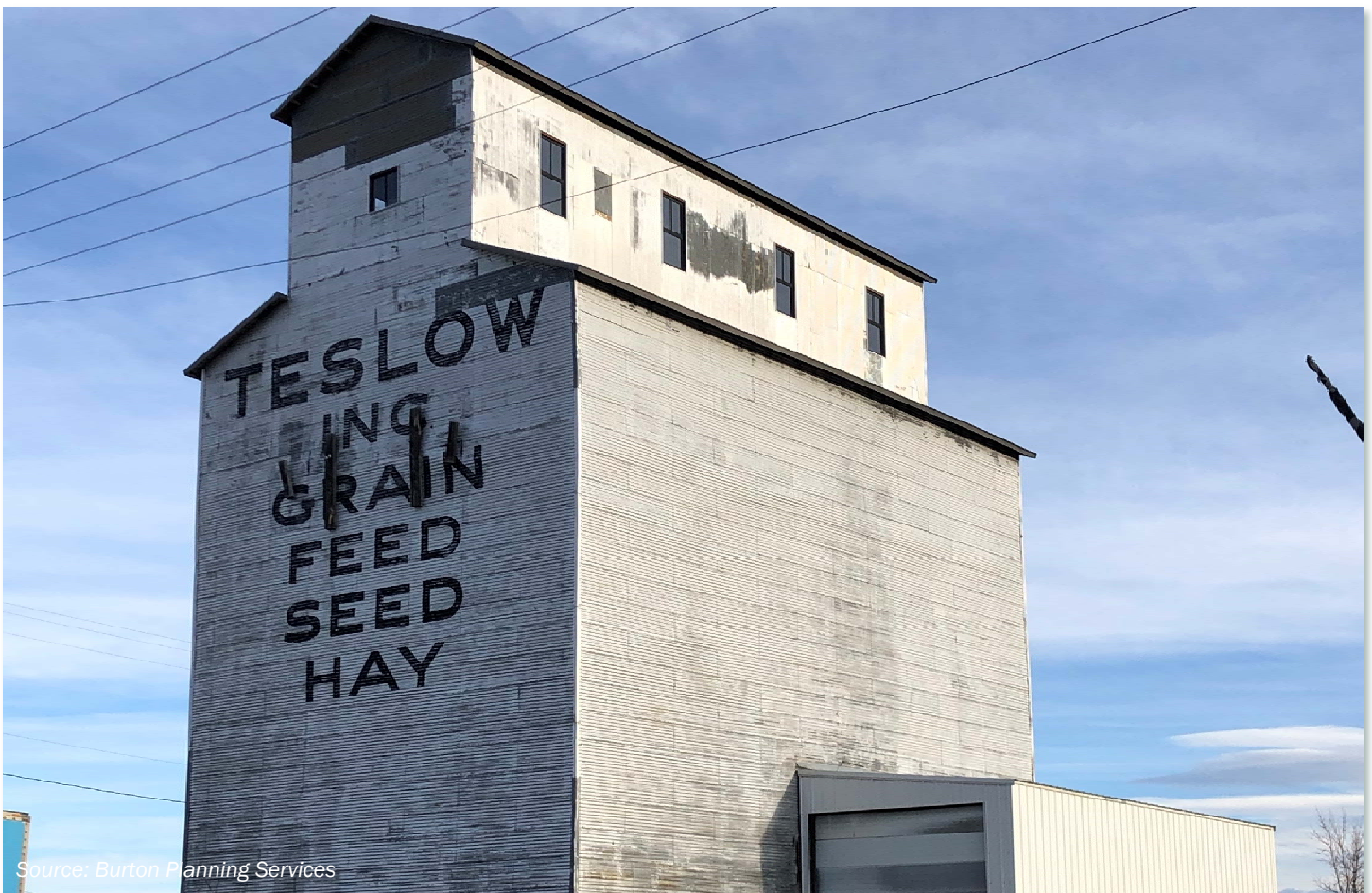
Figure 3.3: Teslow Grain Elevator
