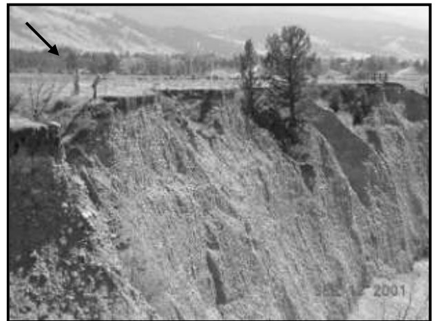
Photo 36. The Weeping Wall. Photo courtesy of DNRC.
