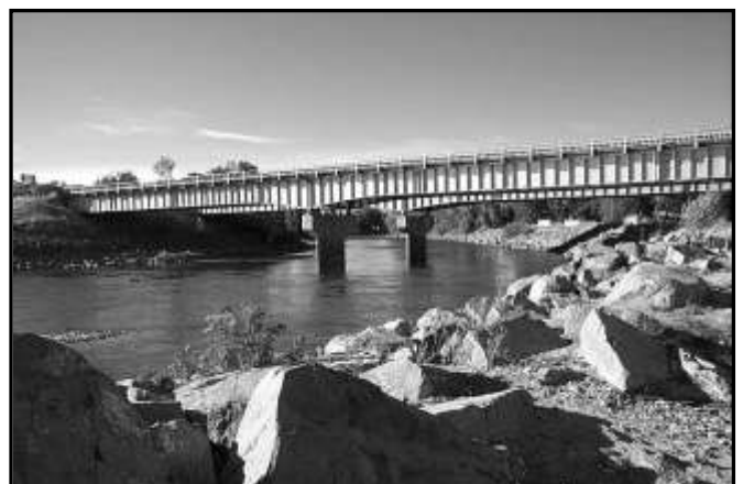
Photo 13. Interstate 90 Bridge. Photo by E. Galli-Noble.
