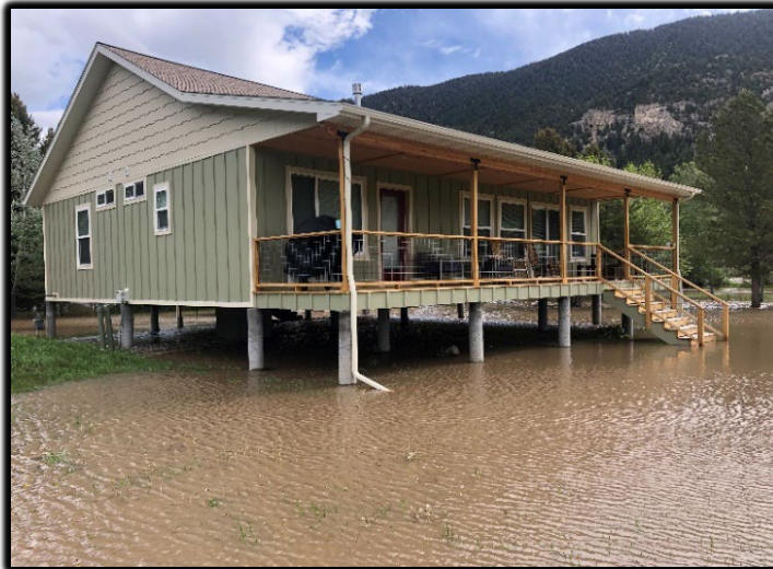
Caption: A residence built along Evergreen Lane off of Highway 89 South near Carter Bridge during and after the 2022 flooding. The residence is located on the banks of the Yellowstone River and avoided inundation due to being built on stilts. Source: Park County.
