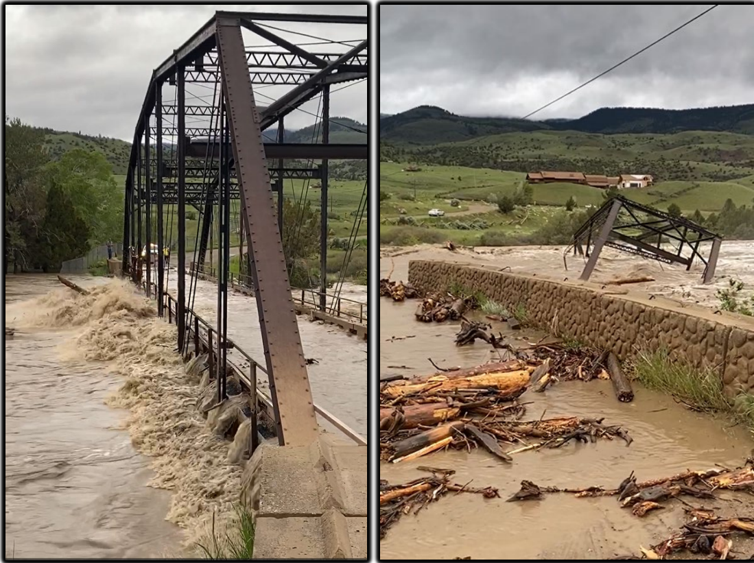
Caption: Carbella Bridge during the 2022 Yellowstone River flood before and during being washed away. Source: Park County.
