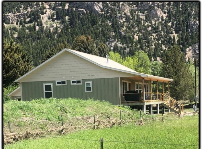
Caption: A residence built along Evergreen Lane off of Highway 89 South near Carter Bridge during and after the 2022 flooding. The residence is located on the banks of the Yellowstone River and avoided inundation due to being built on stilts. Source: Park County.
