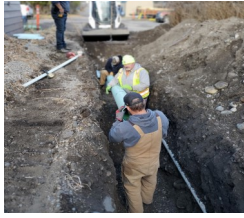
Sewer main project
