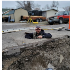
Ryan preparing the corner
