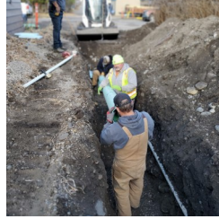
Installing the new pipe
