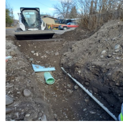
New 8-Inch Insulated Main
