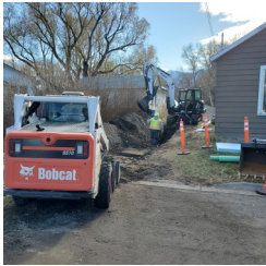
Excavating for new pipe
