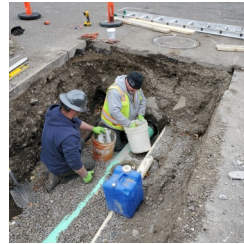
Grouting the new line
