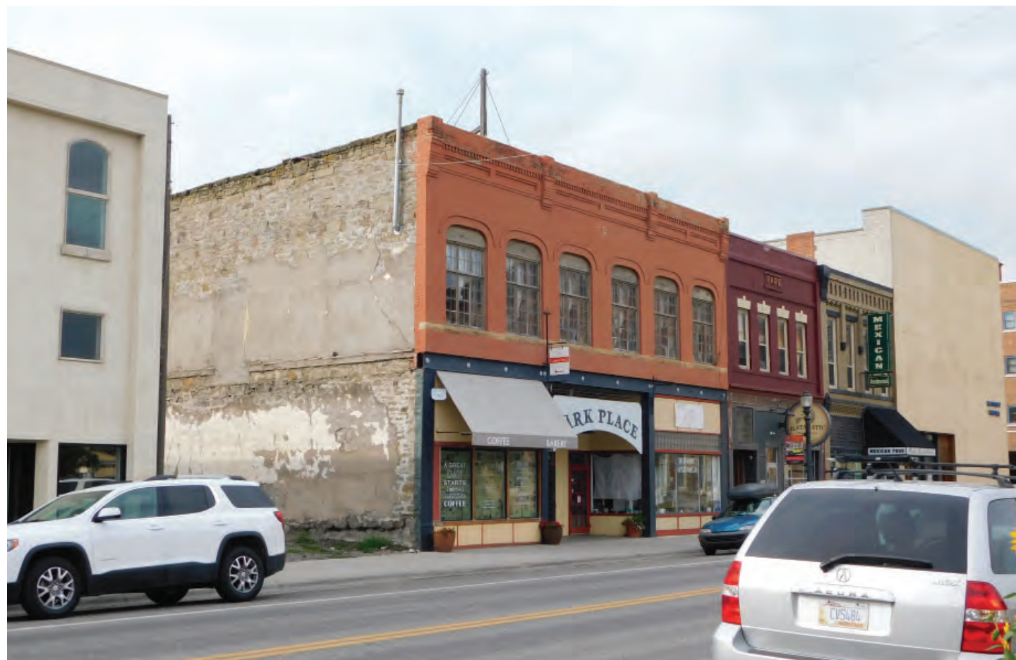
3.4 - Park Place Building Upper Level
